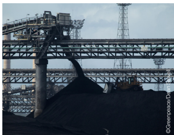
Abbot Point Coal Port Expansion in North Queensland
